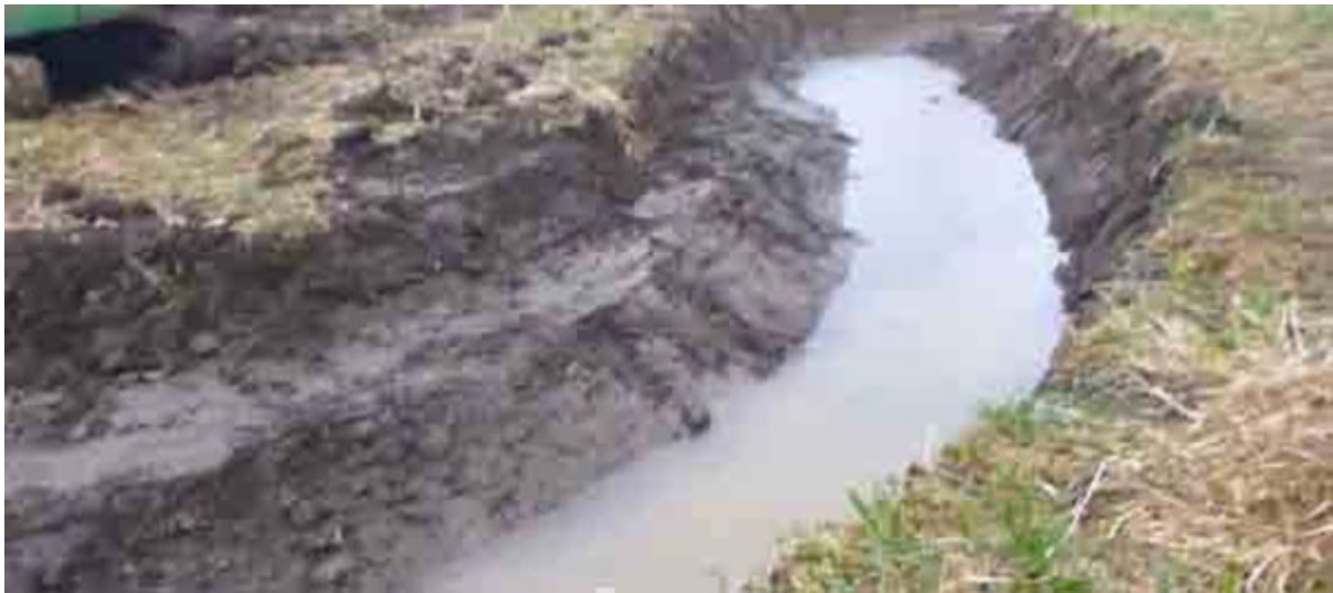
Plate 10 – Example of stepped bend of river bend
